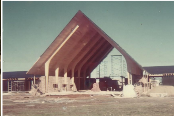
The sanctuary under construction.
