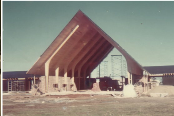
The sanctuary under construction.
