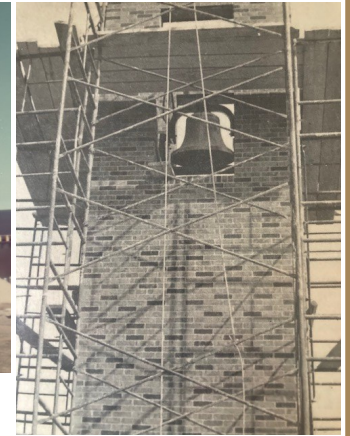
Placing the Bell in its new home.
