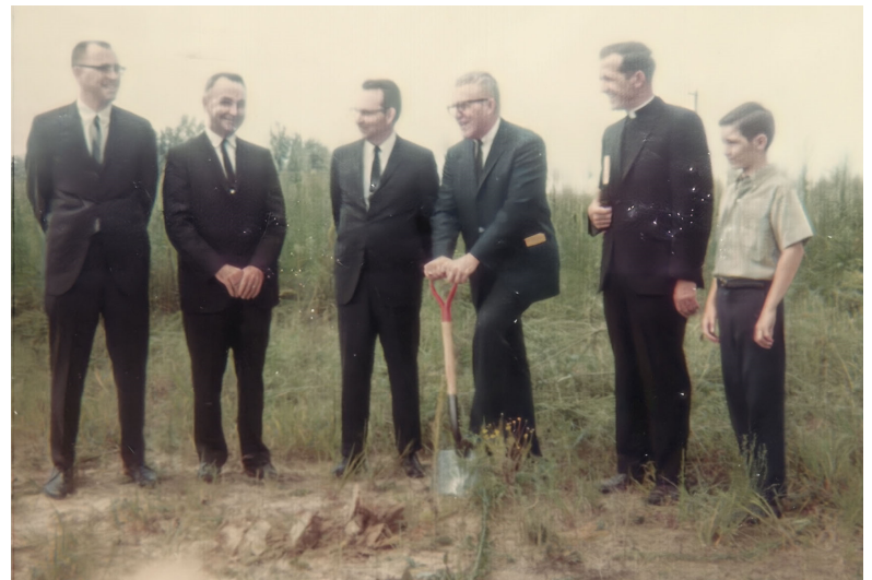
Groundbreaking on Carridale St SW - can you name these fellas?
